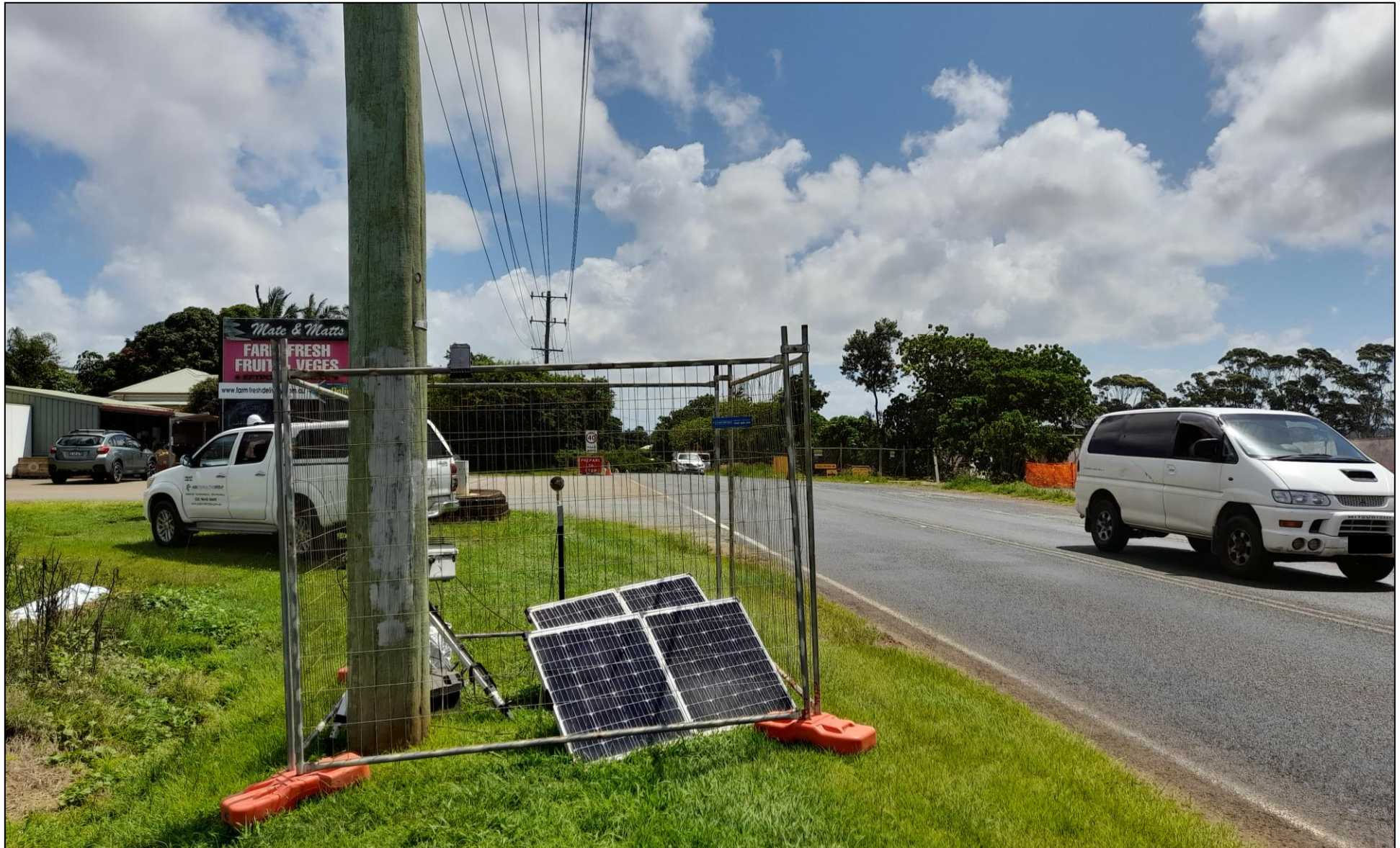
Photograph 3 Representative photograph of monitoring location 006 – Mate and Matts, as observed 06/01/2022
