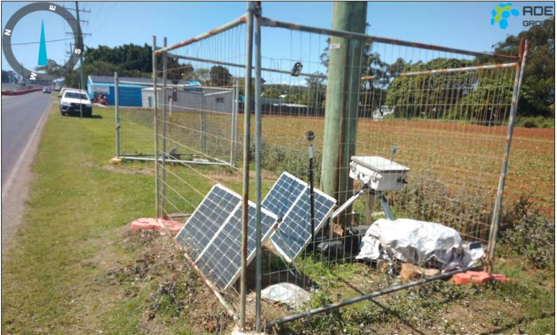
Photograph 3 Representative photograph of monitoring location 006 – Mate and Matts, as observed 12/10/2022
