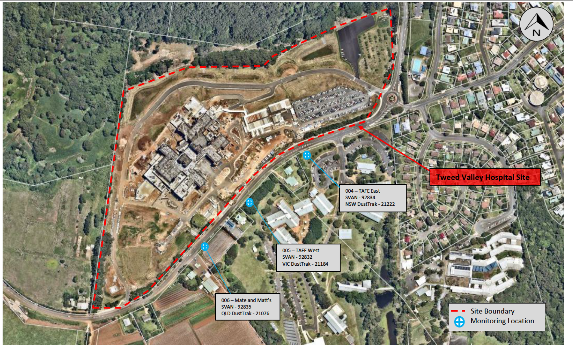
Aerial photograph of the Tweed Valley Hospital Project at Cudgen, NSW (as of 15 th November 2021).
