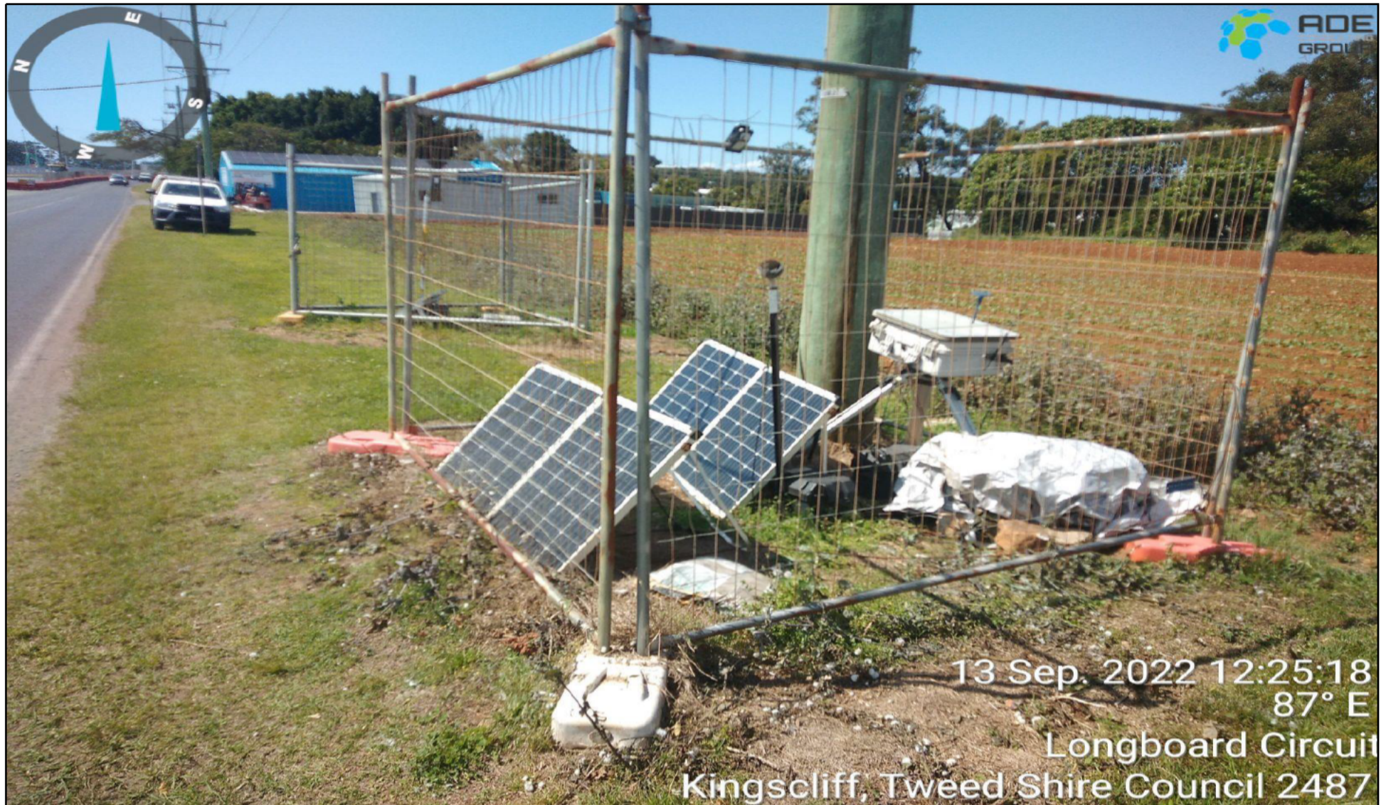
Photograph 3 Representative photograph of monitoring location 006 – Mate and Matts, as observed 13/09/2022
