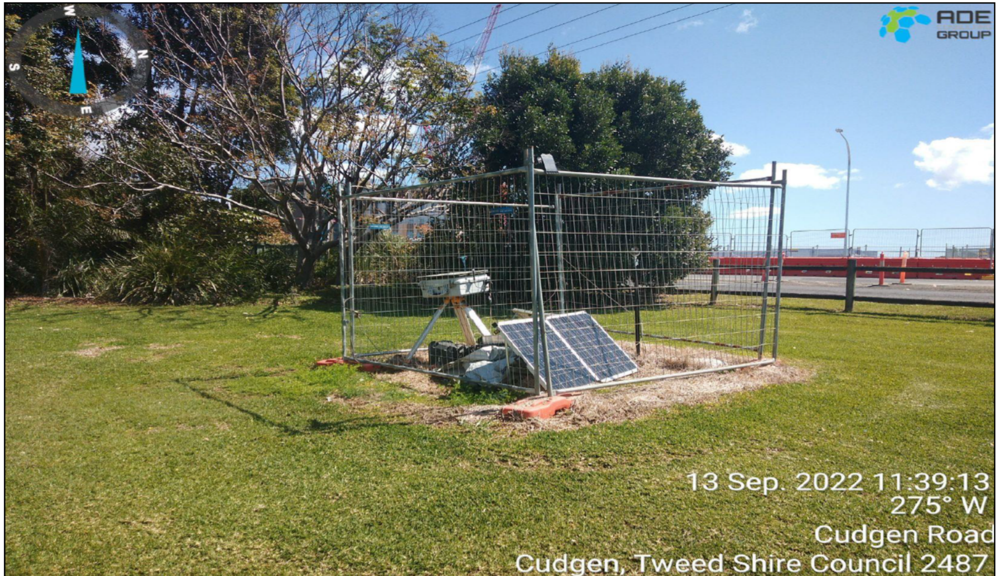
Photograph 1 Representative photograph of monitoring location 004 – TAFE East, as observed 13/09/2022
