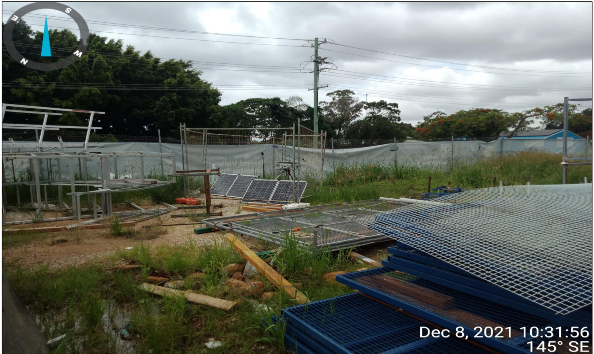
Photograph 1 Representative photograph of monitoring location 001 – Adjacent Carpark location, as observed 08/12/2021
