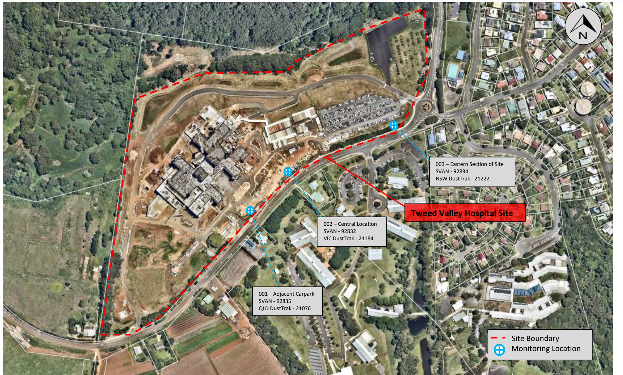
Aerial photograph of the Tweed Valley Hospital Project at Cudgen, NSW (as of 15 November 2021).
