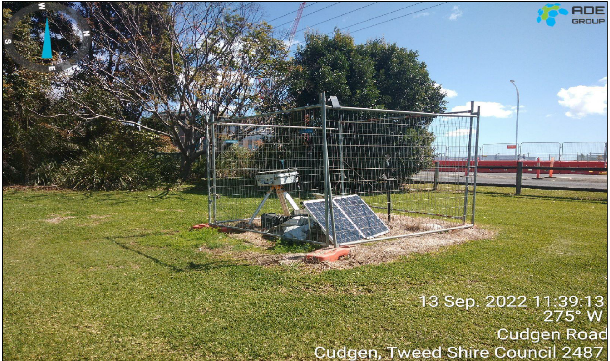
Photograph 1 Representative photograph of monitoring location 004 – TAFE East, as observed 13/09/2022
