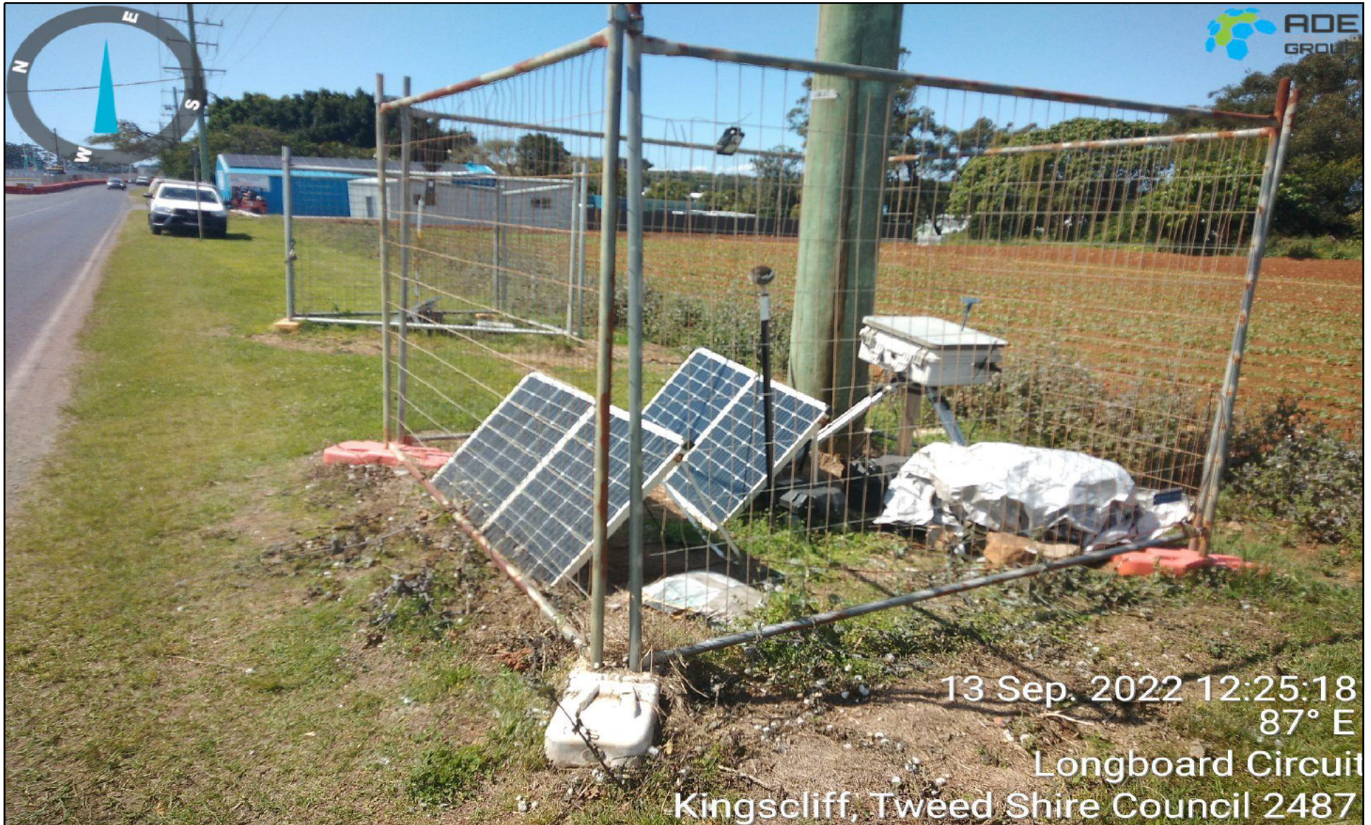
Photograph 3 Representative photograph of monitoring location 006 – Mate and Matts, as observed 13/09/2022
