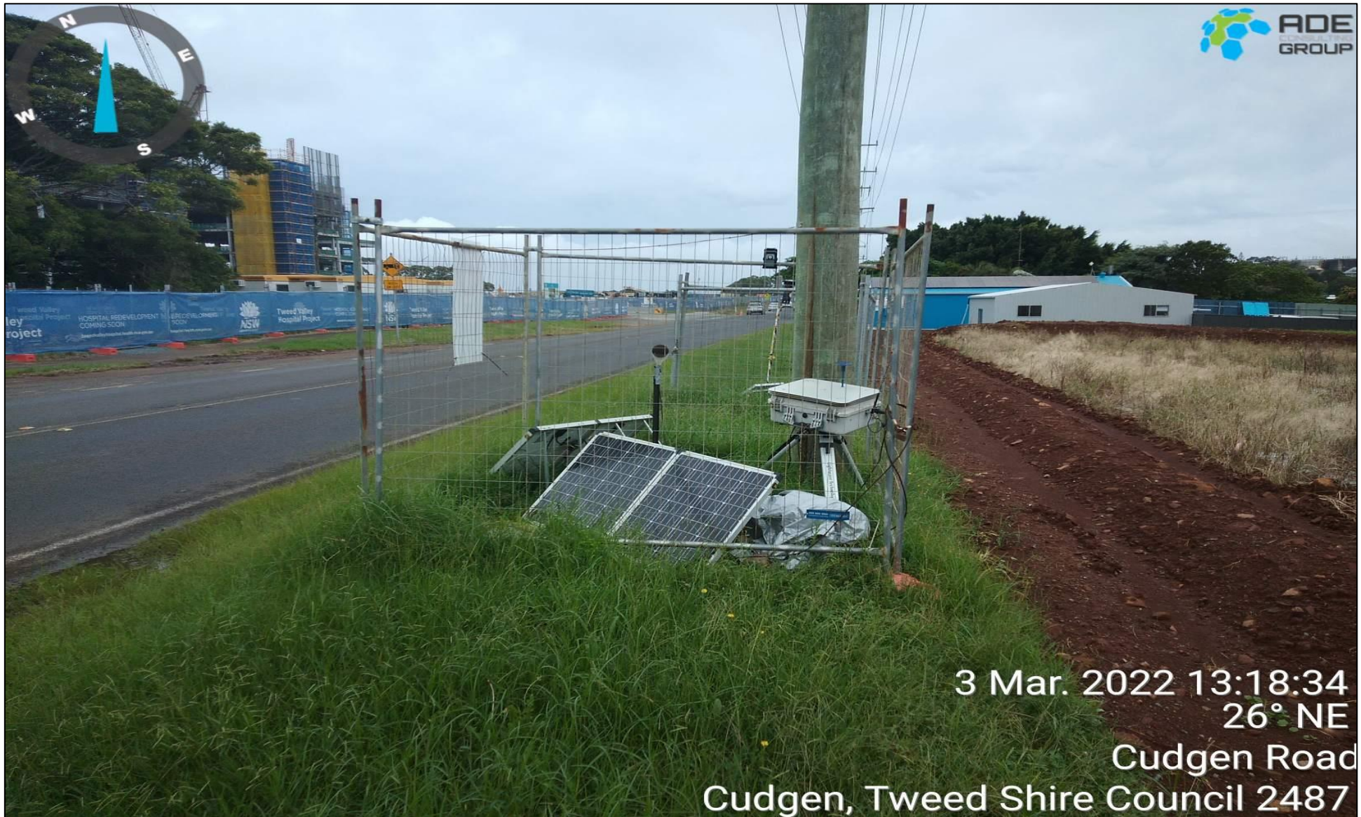
Photograph 3 Representative photograph of monitoring location 006 – Mate and Matts, as observed 03/03/2022
