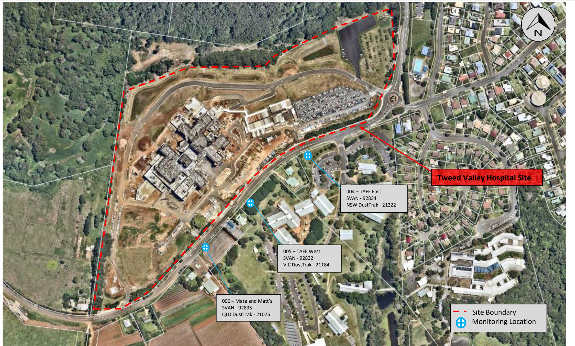
Aerial photograph of the Tweed Valley Hospital Project at Cudgen, NSW (as of 15 th November 2021).
