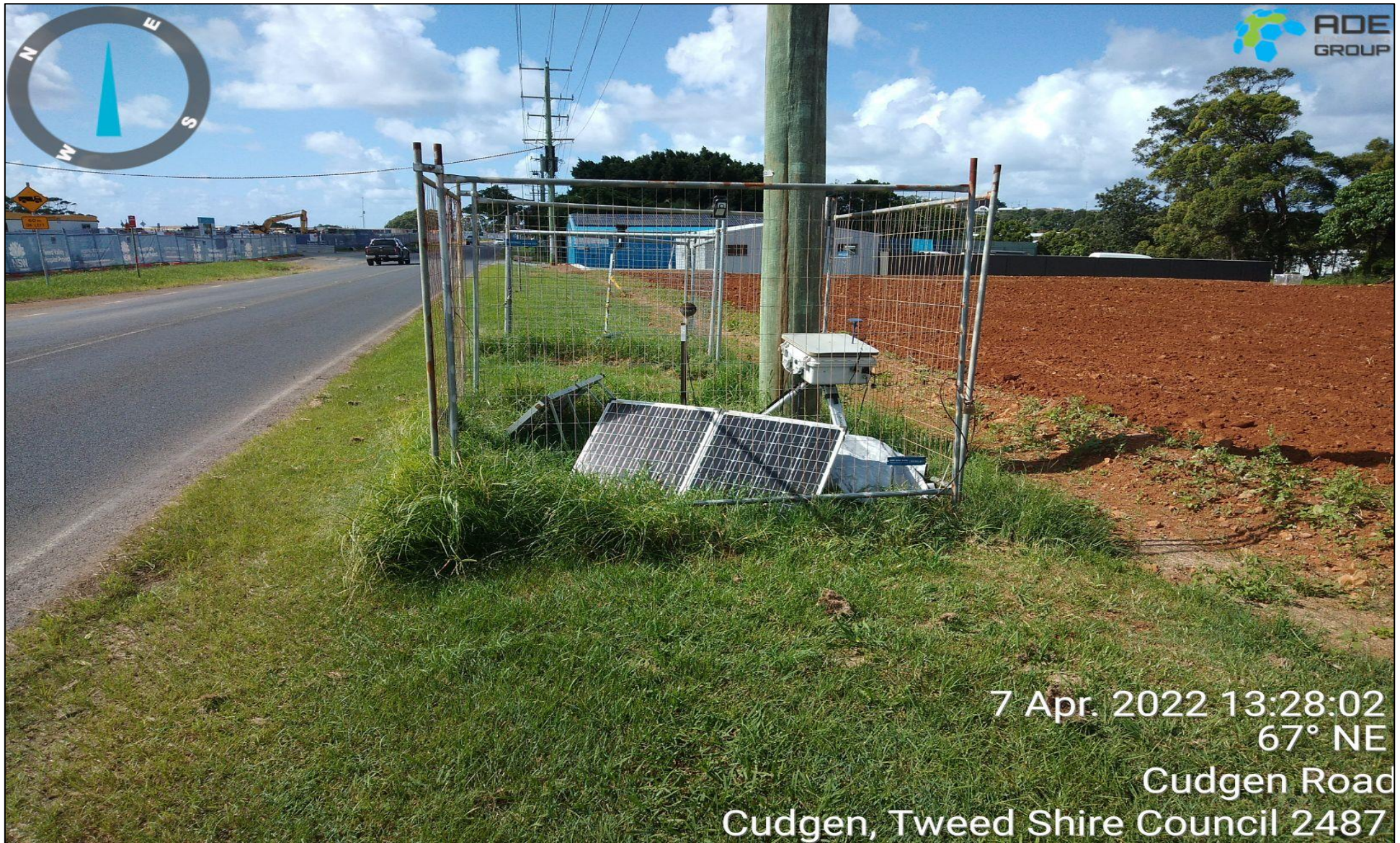
Photograph 3 Representative photograph of monitoring location 006 – Mate and Matts, as observed 07/04/2022
