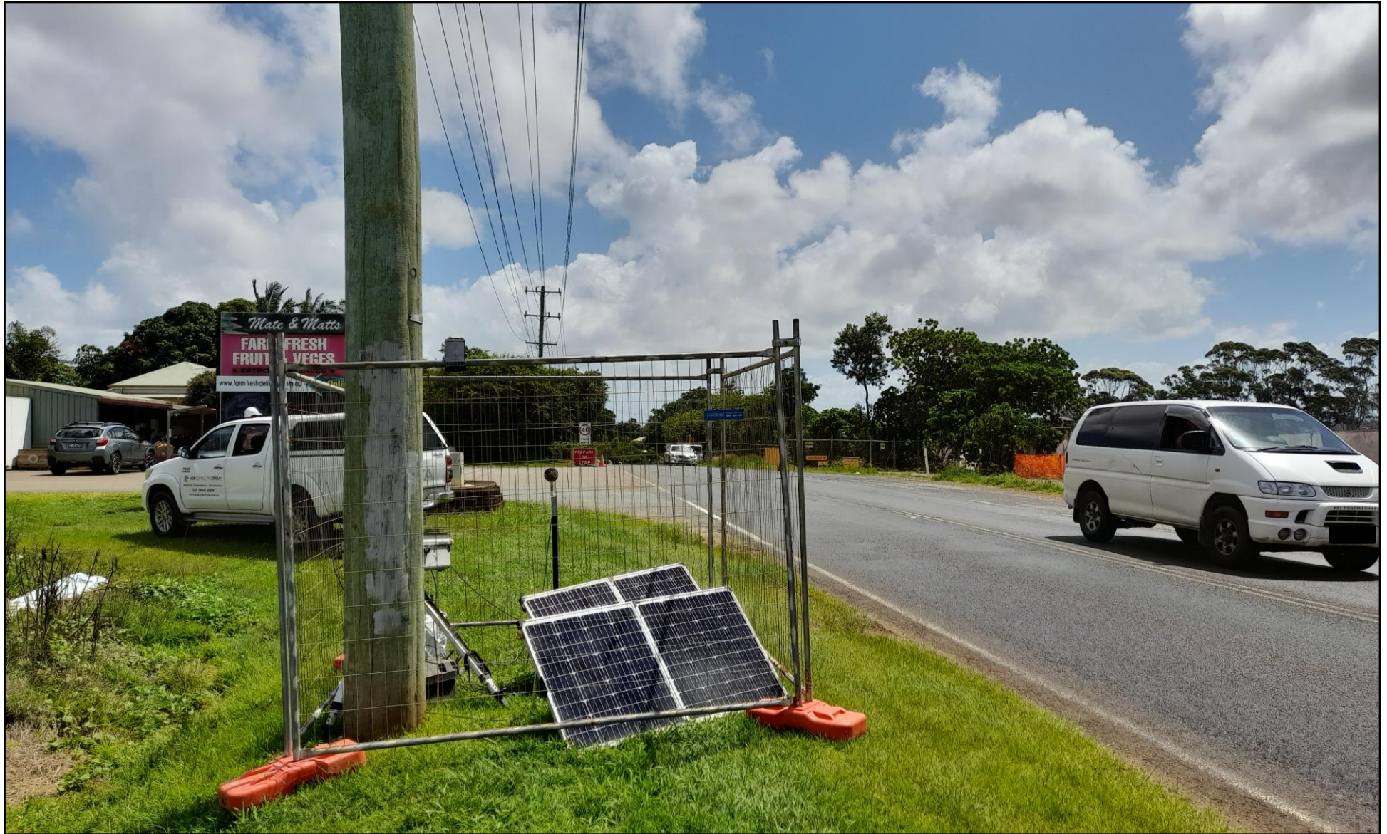
Photograph 3 Representative photograph of monitoring location 006 – Mate and Matts, as observed 11/01/2022
