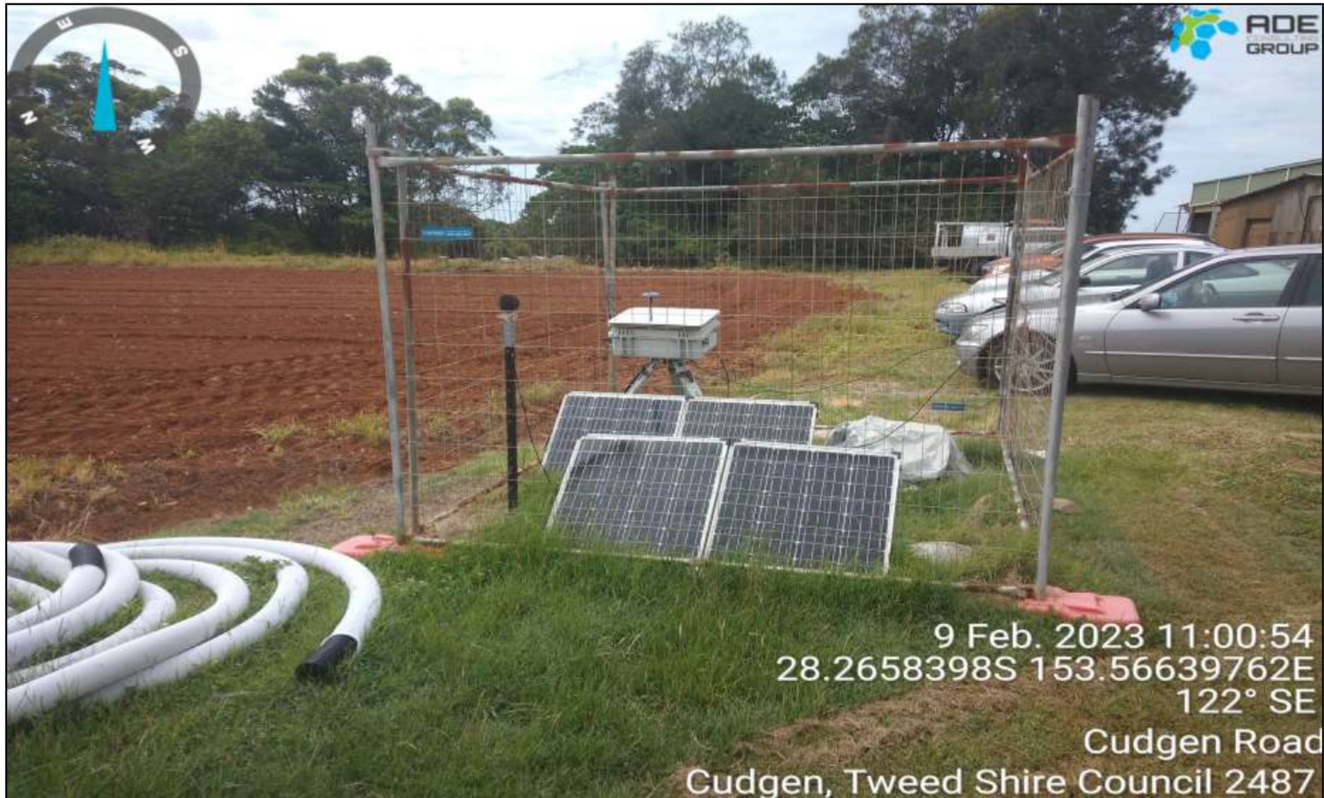
Photograph 3 Representative photograph of monitoring location 006 – Mate and Matts, as observed 09/02/2023
