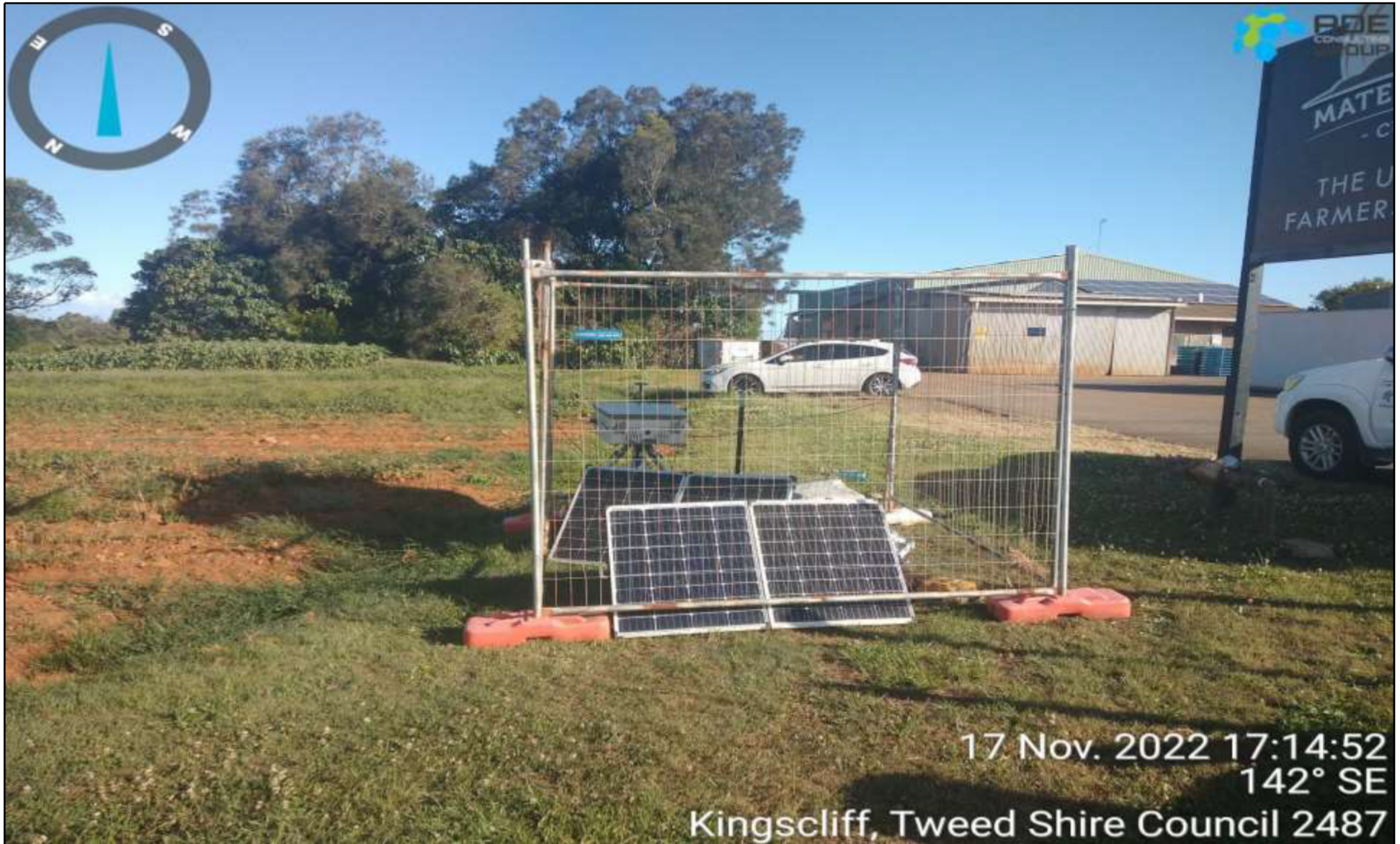
Photograph 3 Representative photograph of monitoring location 006 – Mate and Matts, as observed 17/11/2022
