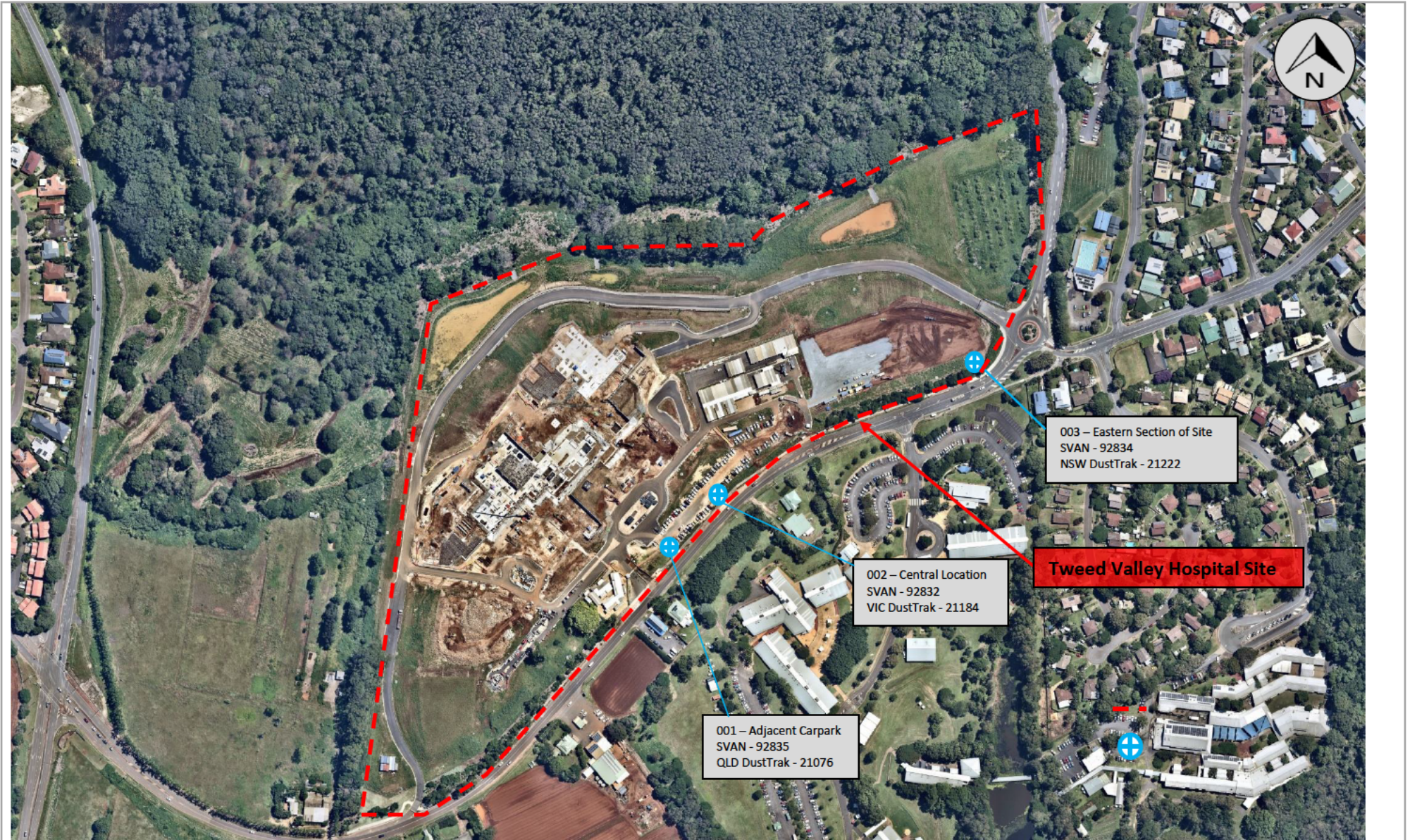
Aerial photograph of the Tweed Valley Hospital Project at Cudgen, NSW (as of 5 th of March 2021).
