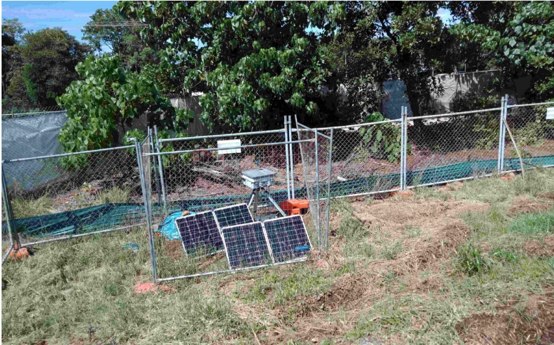
Photograph 3 Representative photograph of monitoring location 003 – Eastern Section of Site, as observed 24/03/2021
