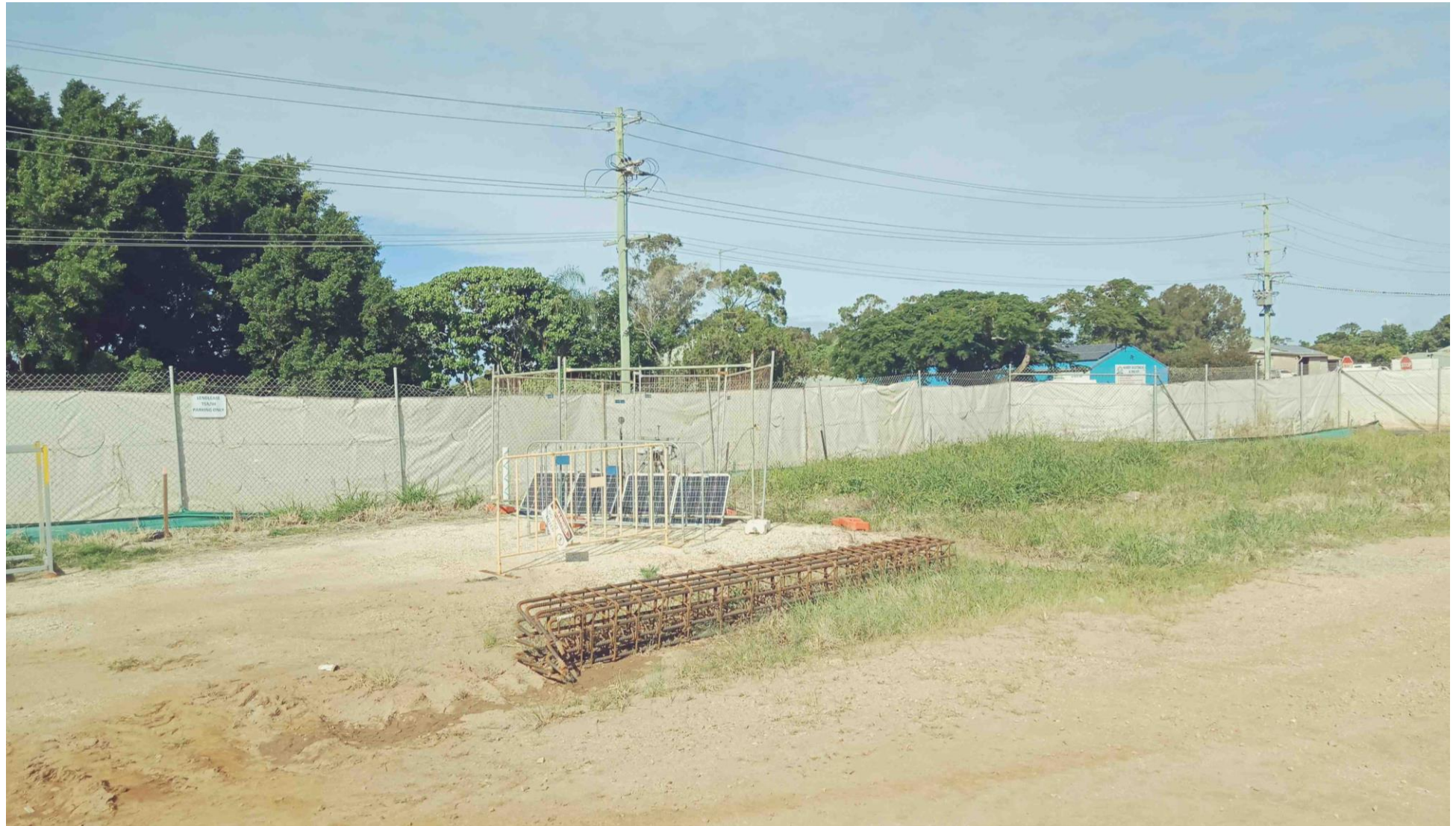
Photograph 1 Representative photograph of monitoring location 001 – Adjacent Carpark location, as observed 01/06/2021
