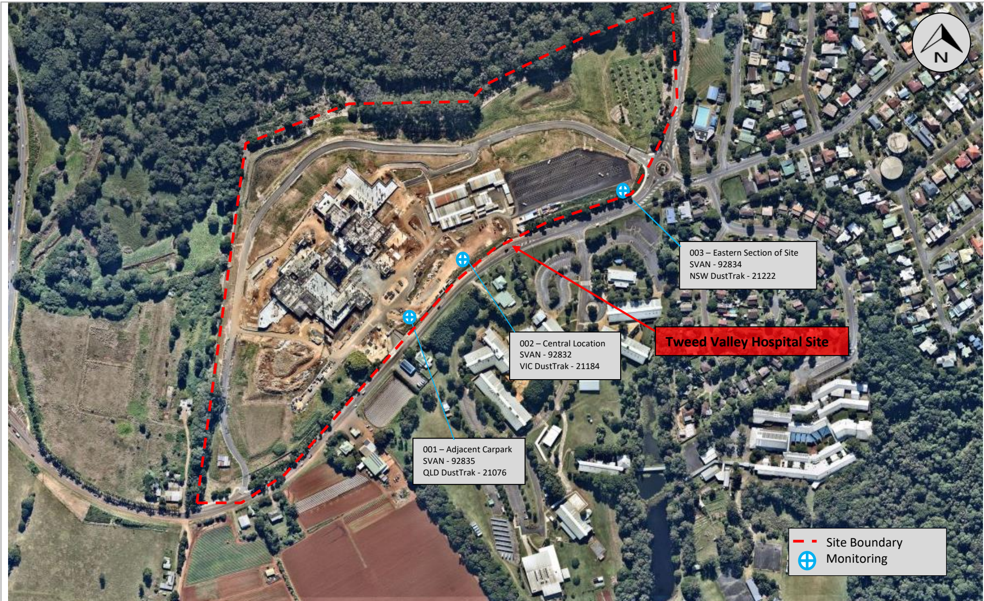
Aerial photograph of the Tweed Valley Hospital Project at Cudgen, NSW (as of 6 th of June 2021).
