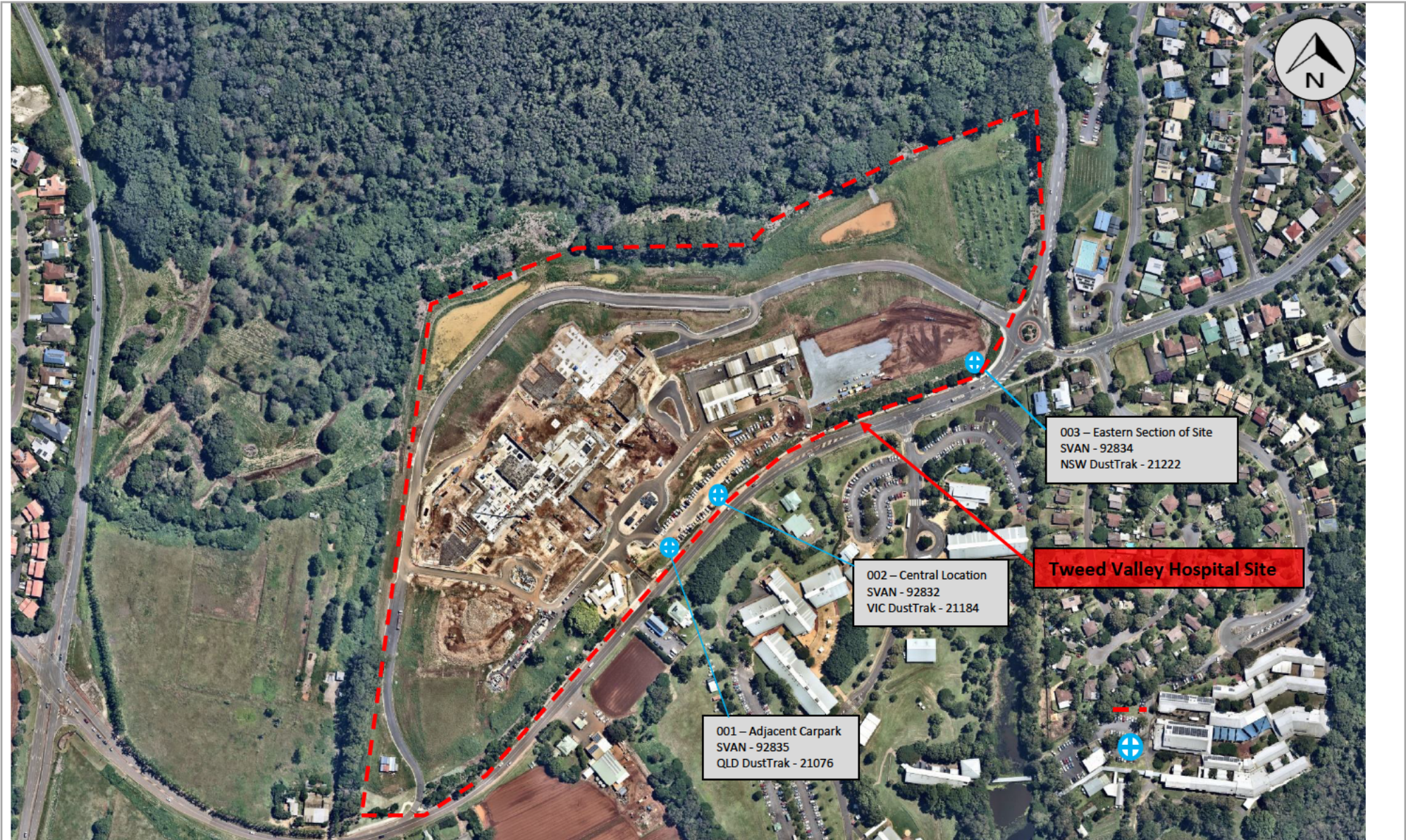
Aerial photograph of the Tweed Valley Hospital Project at Cudgen, NSW (as of 5 th of March 2021).
