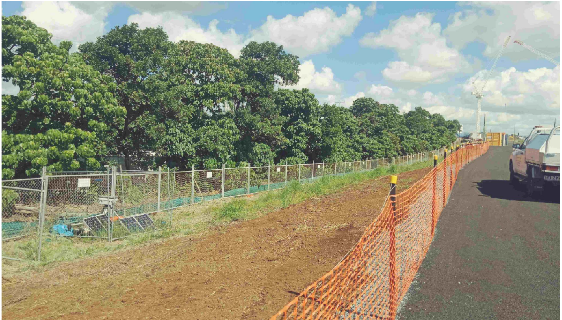
Photograph 3 Representative photograph of monitoring location 003 – Eastern Section of Site, as observed 27/04/2021
