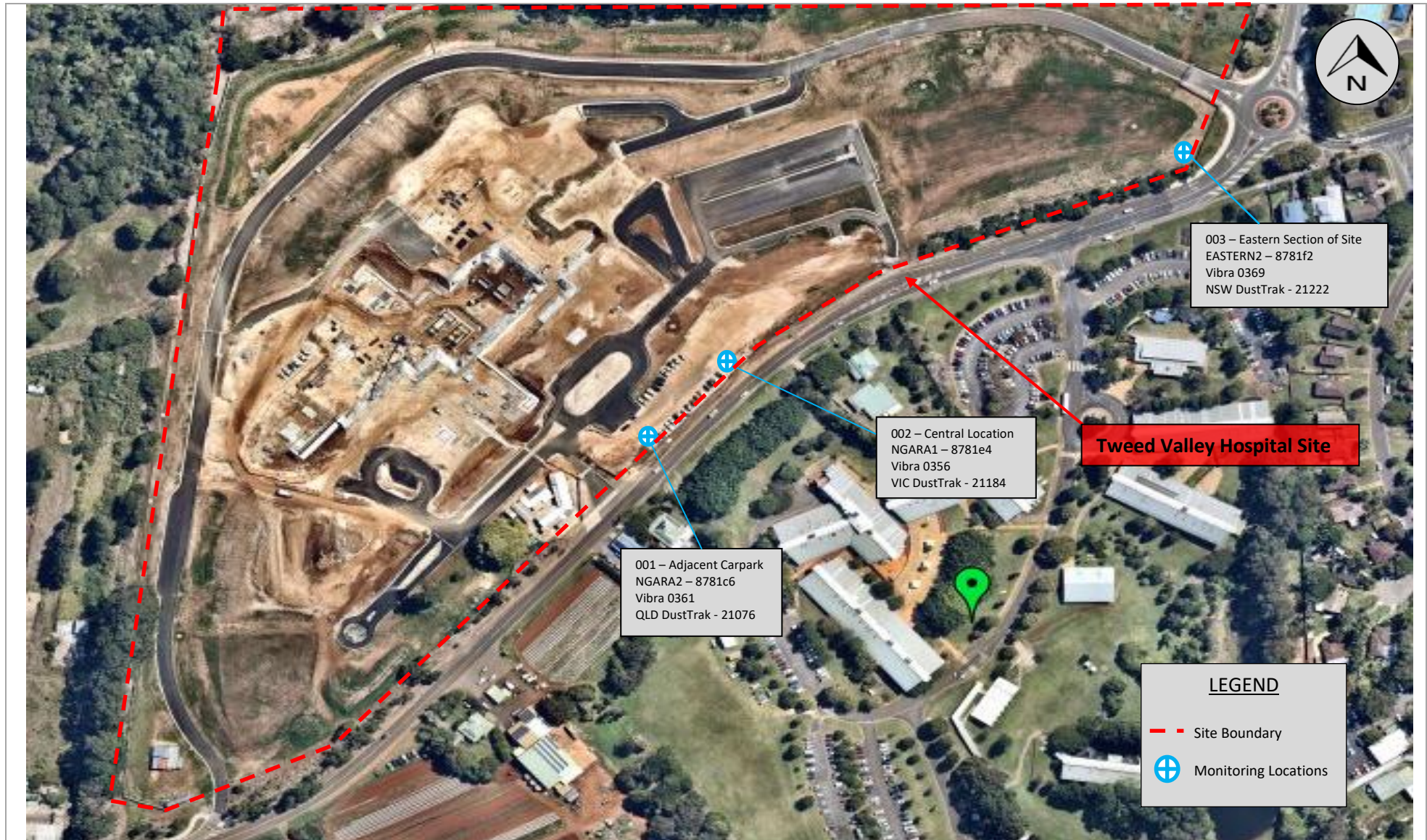
Aerial photograph of the Tweed Valley Hospital Project at Kingscliff, NSW (as of 30 November 2020).
