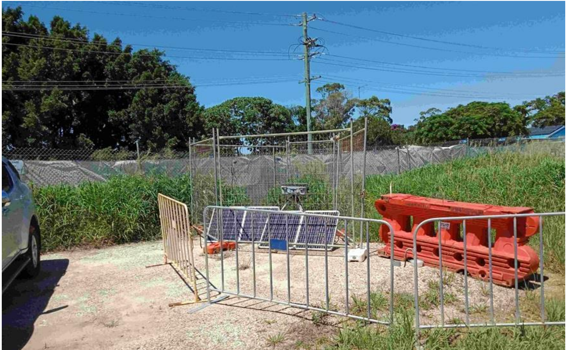
Photograph 1. Representative photograph of monitoring location 001 – Adjacent Carpark location, as observed 22/02/21.
