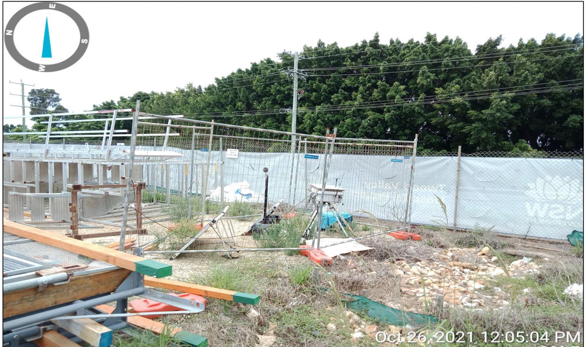
Photograph 1 Representative photograph of monitoring location 001 – Adjacent Carpark location, as observed 26/10/2021
