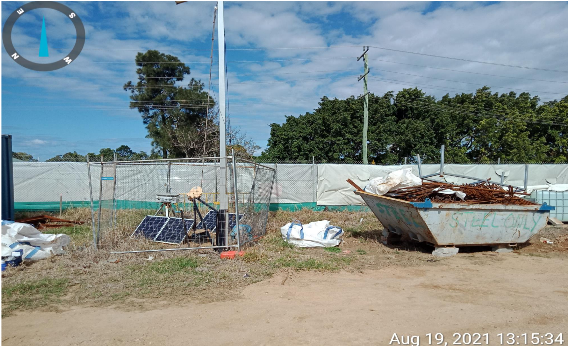
Photograph 2 Representative photograph of monitoring location 002 – Central location, as observed 19/08/2021
