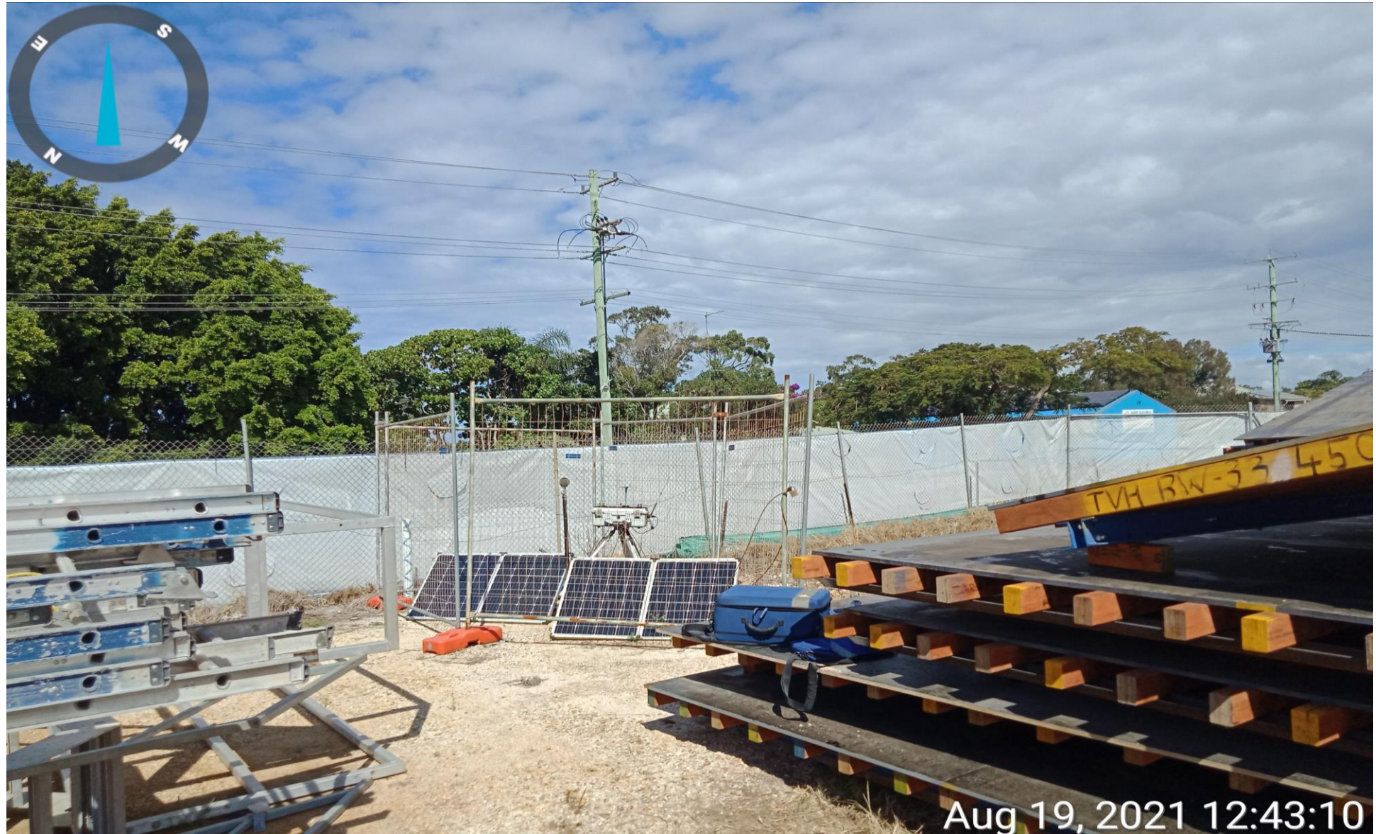
Photograph 1 Representative photograph of monitoring location 001 – Adjacent Carpark location, as observed 19/08/2021
