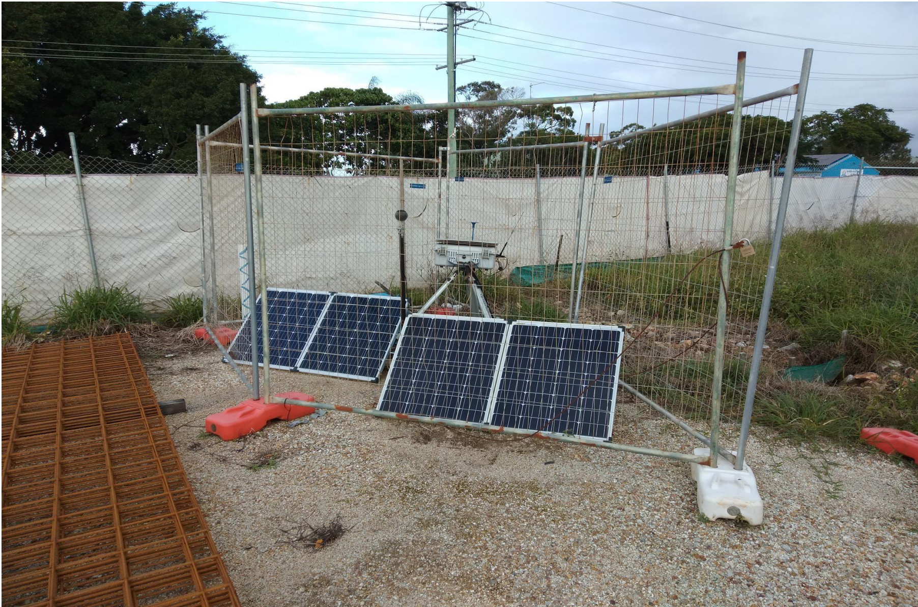
Photograph 1 Representative photograph of monitoring location 001 – Adjacent Carpark location, as observed 02/07/2021
