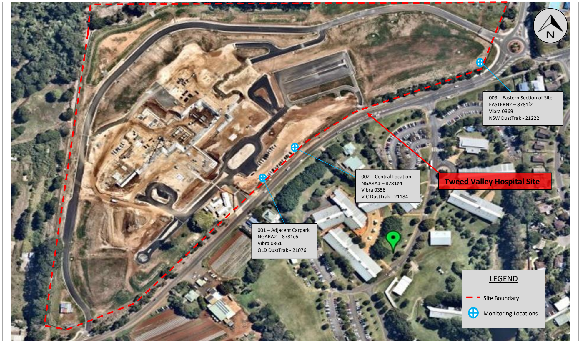
Aerial photograph of the Tweed Valley Hospital Project at Kingscliff, NSW (as of 30 November 2020).
