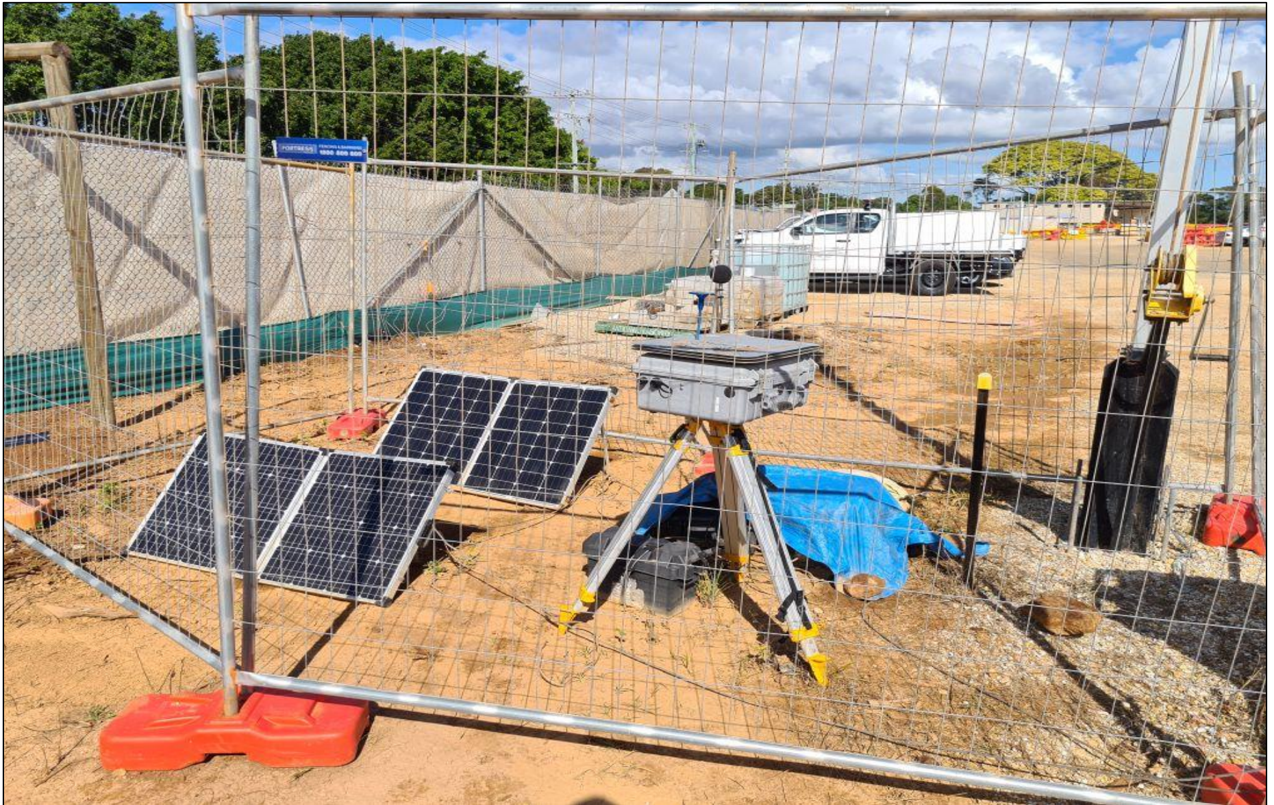
Photograph 2. Representative photo of monitoring location 002 – Central location, as observed 04.08.2020.
