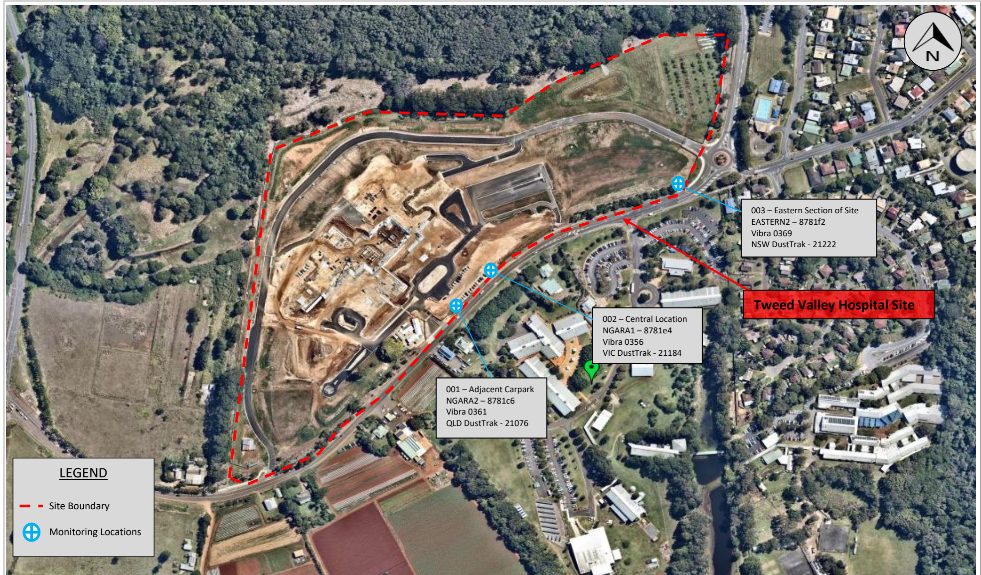
Aerial photograph of the Tweed Valley Hospital Project at Kingscliff, NSW (as of 6 th October 2020).
