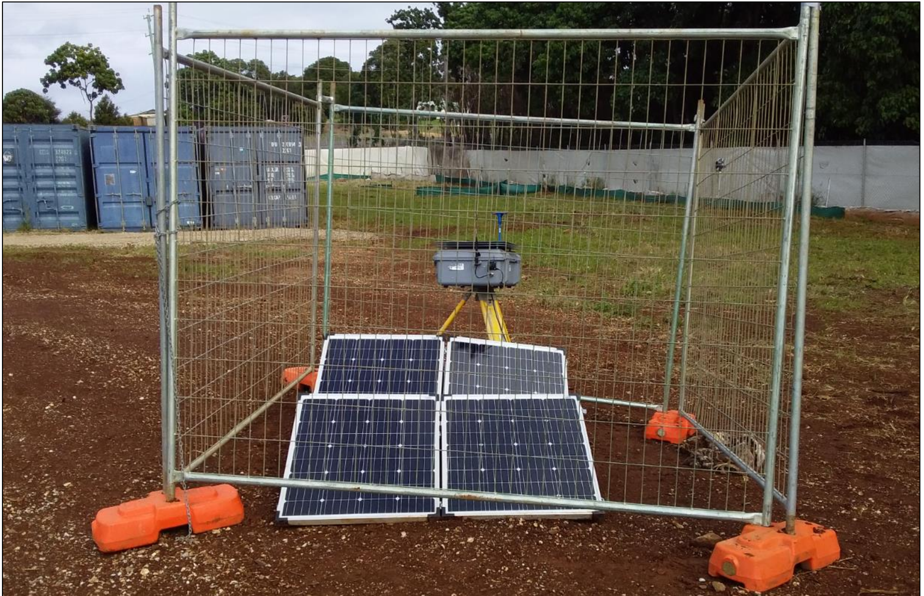
Photograph 6. Representative photo of monitoring location 006 – South Western Dust Monitor, as observed 18.06.2020.
