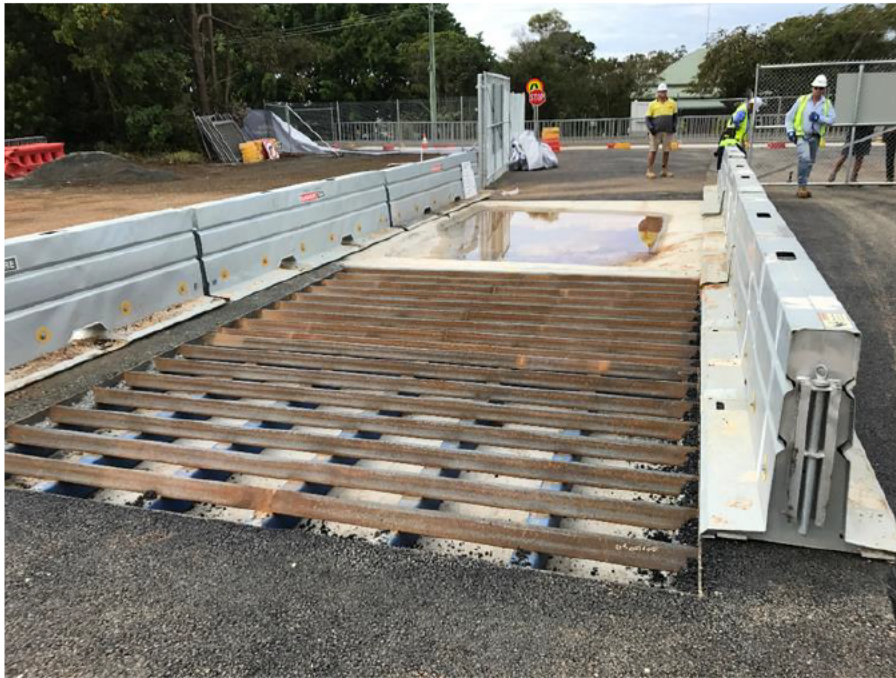
Figure 5 Rumble grid and wheel wash at site exit
