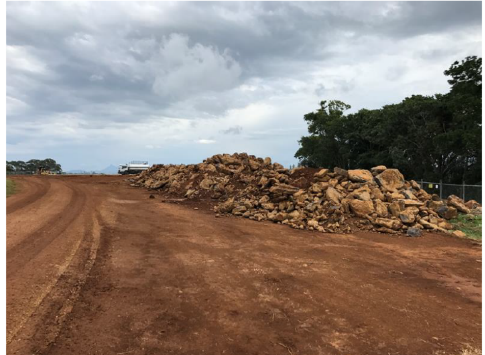
Figure 4 Cleared site with stockpiles
