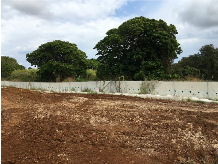
Figure 3 Site fencing with fauna crossing
